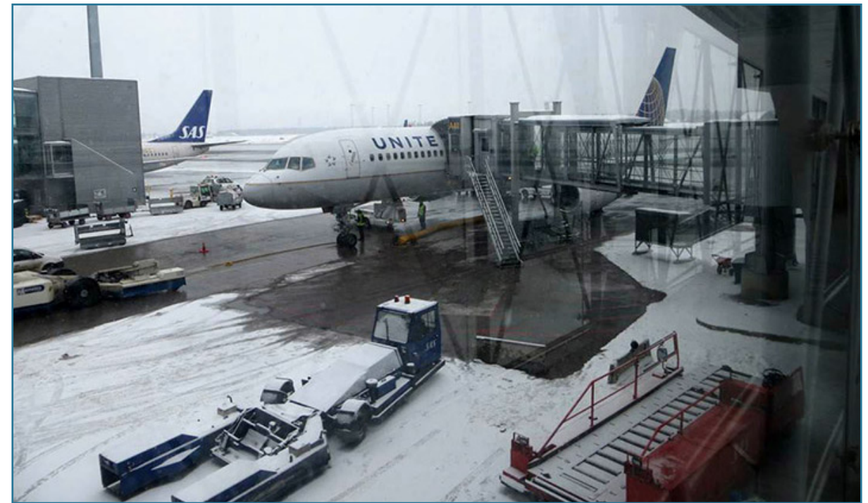
This photo, taken at the airport in Oslo, Norway, shows the potential for heated pavement technology — in this case, geothermal heating. Note the taxiway and gate area are free of snow and ice.
